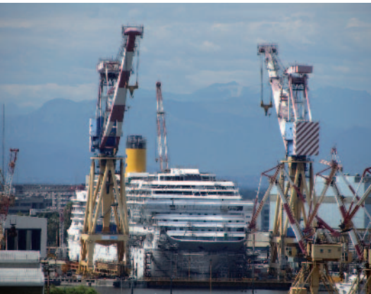
© Waerfelu - Cruise ship under construction at the Porto Marghera shipyard
