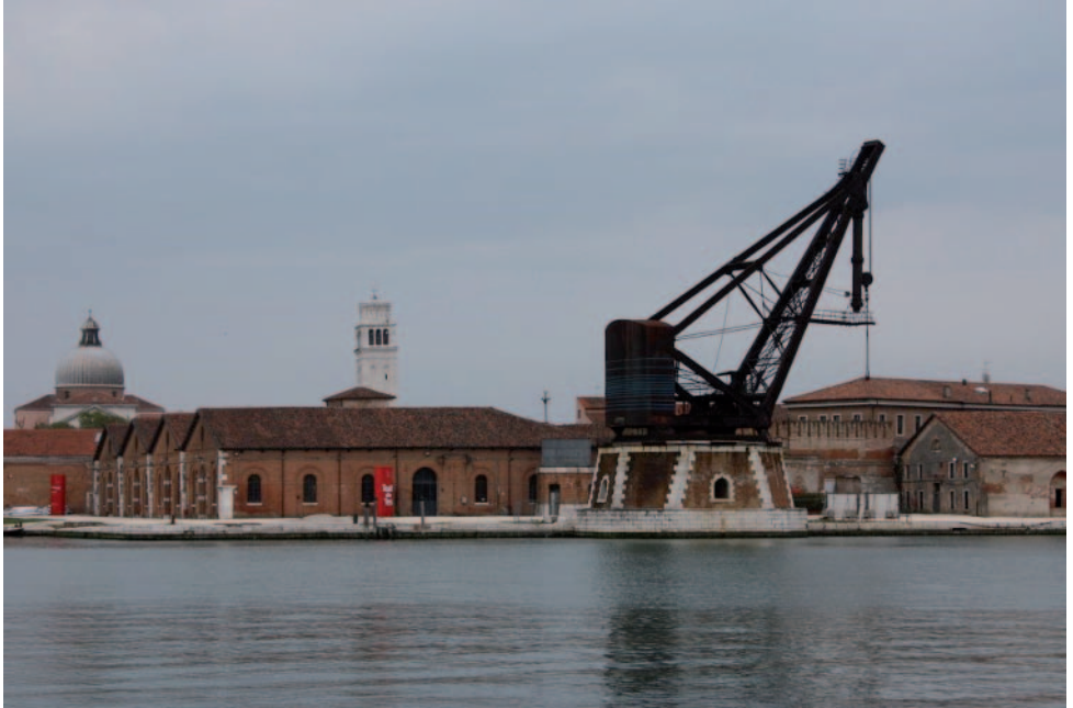
© Martin Wippel · The Darsena Grande with the 19th century Armstrong-Mitchell crane and 16th century warehouses
